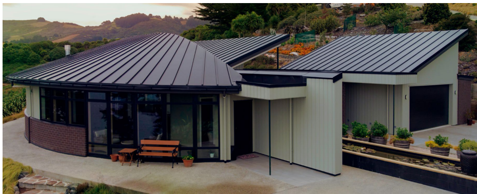
Dimond rainwater system application - fascia, gutter and downpipe installation.
