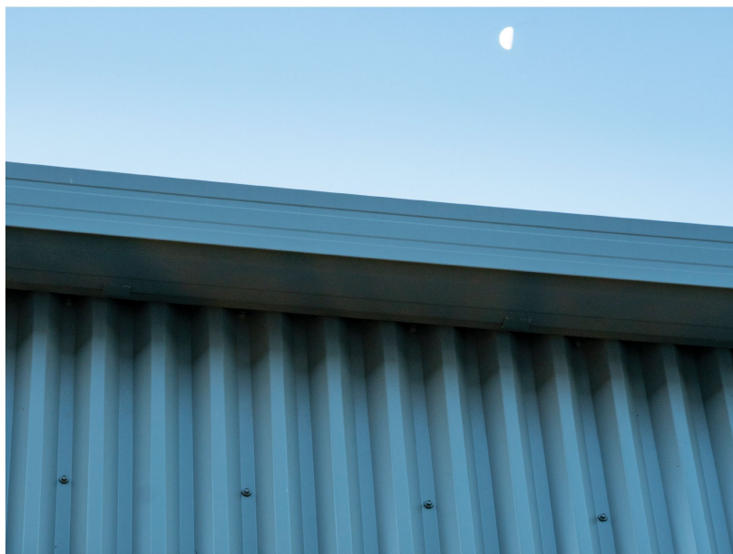
Example of eaves gutter installation with roof cladding and wall cladding below.
